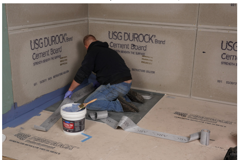
Embedding joint reinforcement tape over floor-to-wall joints.
