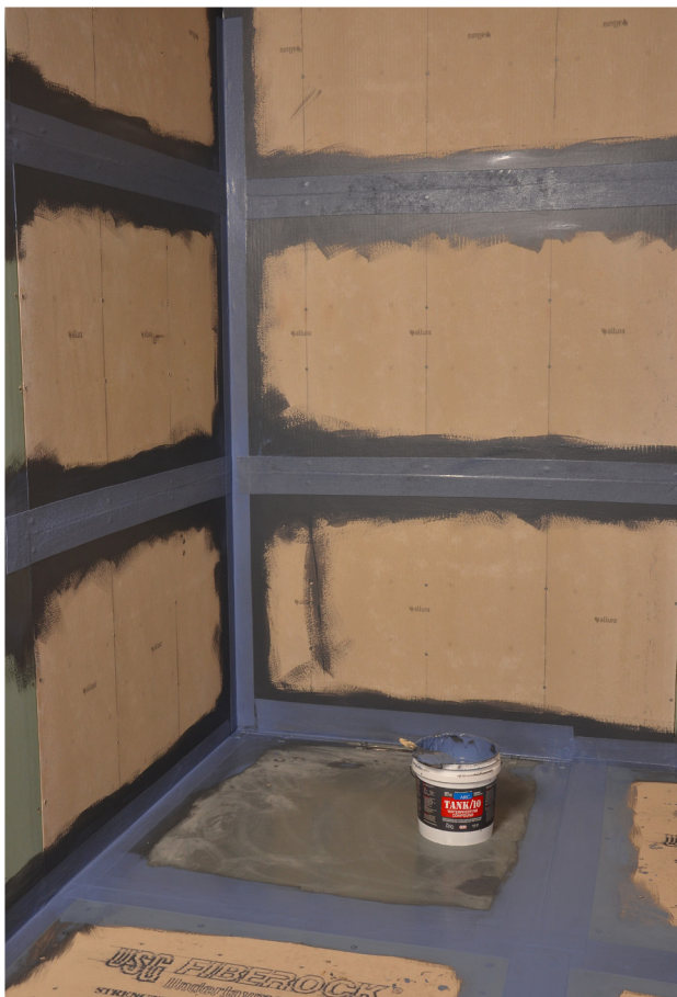
Joint reinforcement tape covering joints in shower area.
